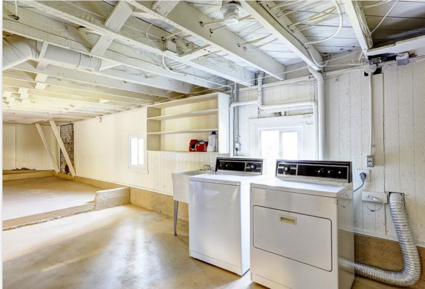
Existing Windows in CONVERTED space
