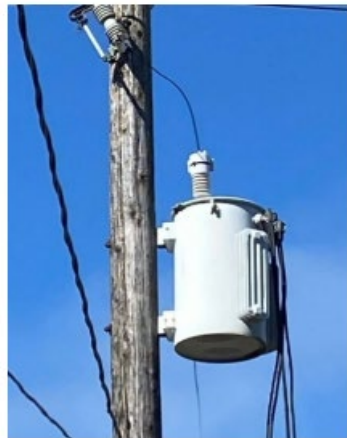
Figure 23. Pole-Mounted Transformer
